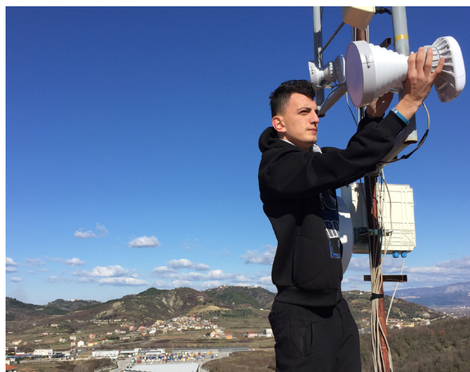
Starnet technician installing RF elements® equipment
